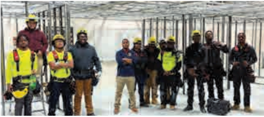
Students from YouthBuild Boston participated in a Shop Friday Intro to Metal Framing class with NASCTF Instructor Decio Santos (center) at the Boston training facility.
