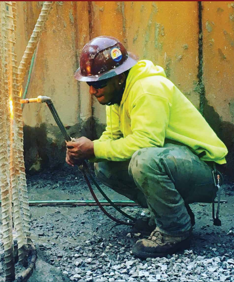
Justin Alves Pile Drivers Local 56
