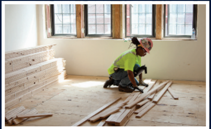
Tasha Wormley of Carpenters Local 24 installs flooring in a dorm room.
