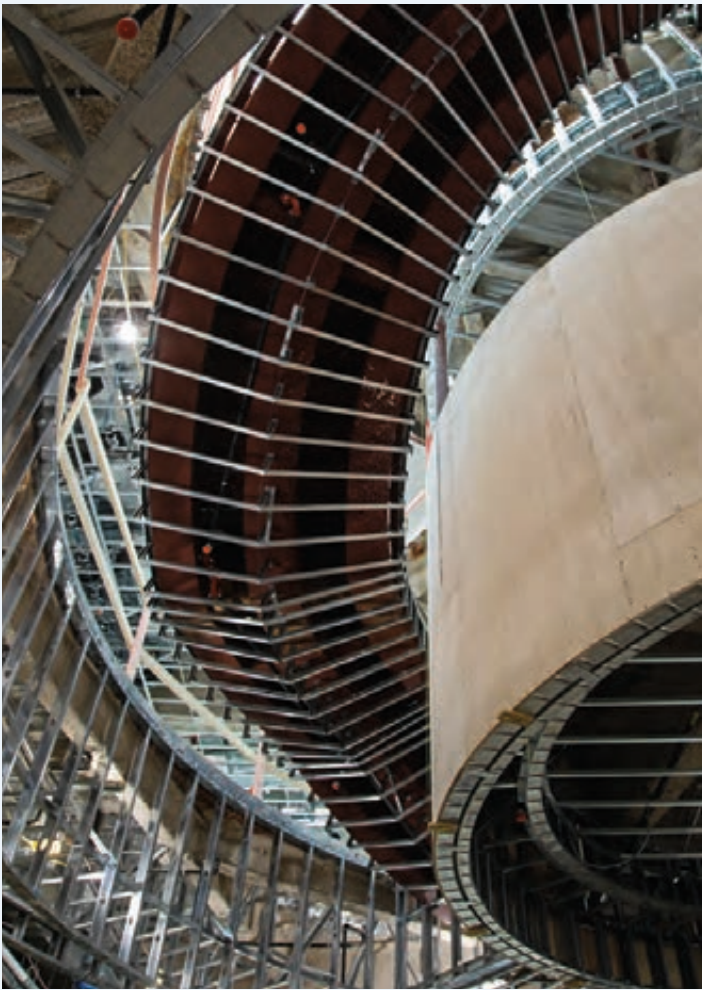
A view of the complex interior systems work of the underside of a full parallel landed spiral grand staircase.
