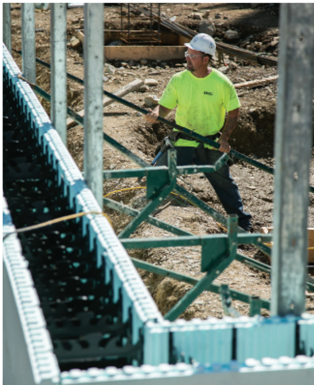
Gary Smith of Woodframe Local 723 installs strongbacks and scaffolding.
